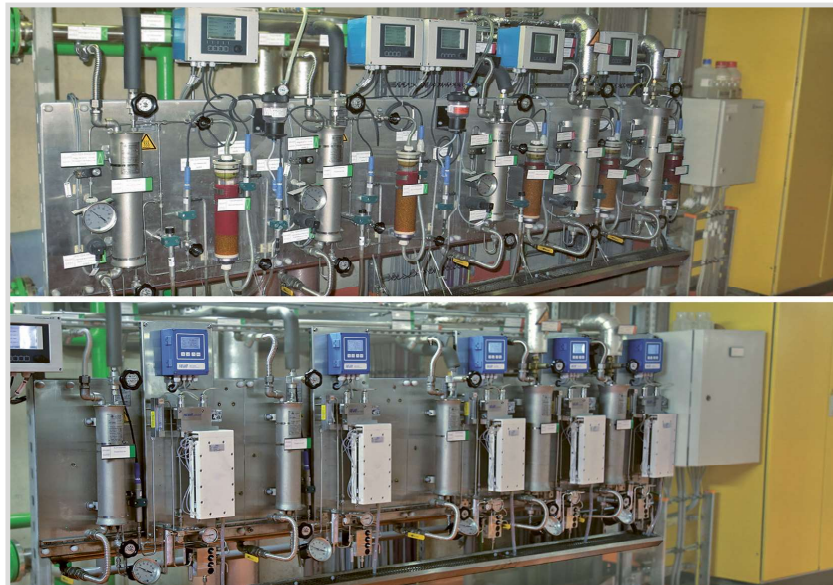
Fig. 7. Main sampling system for feedwater: Before and after.
